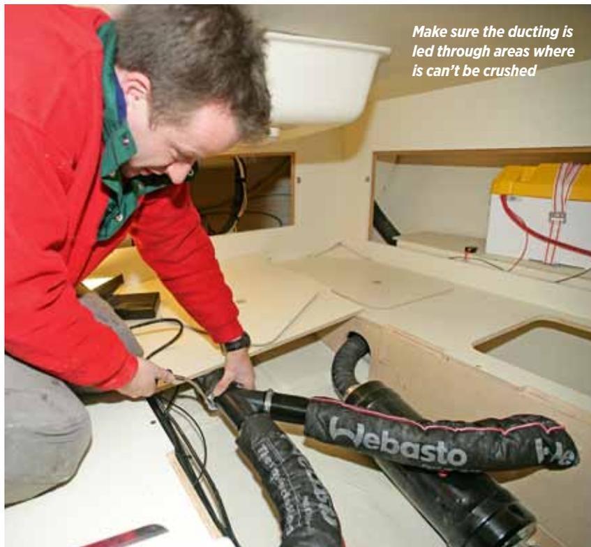
**Make sure the ducting is led through areas where is can't be crushed**
